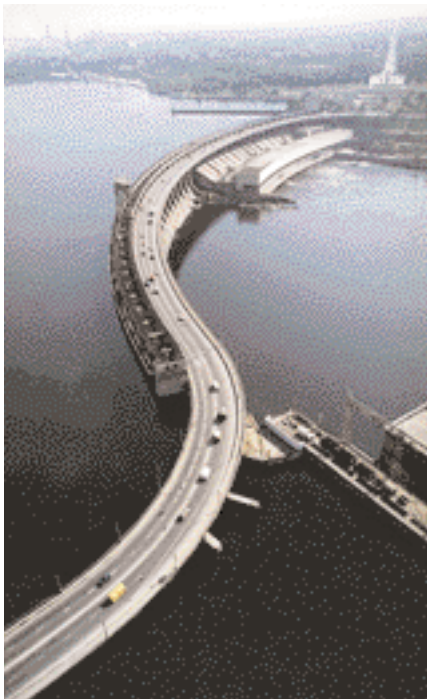
The Dniaprobes Dam in Zaporizhzhia
